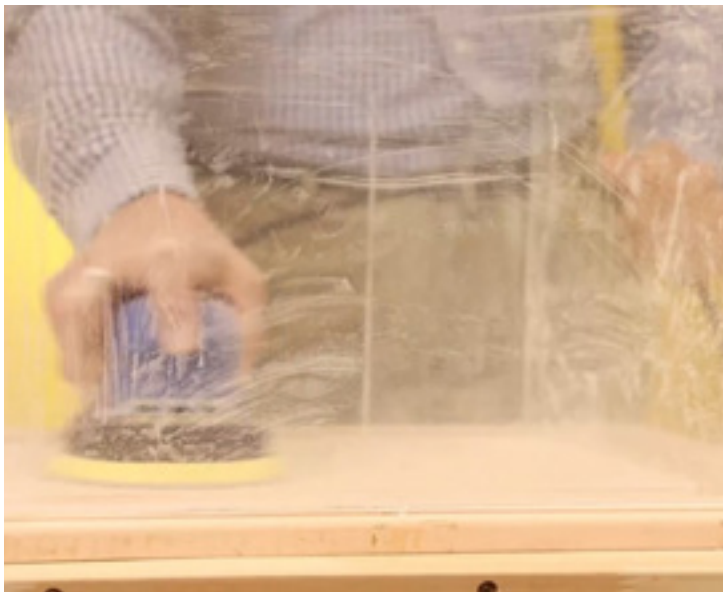
Sanding without dust extraction
